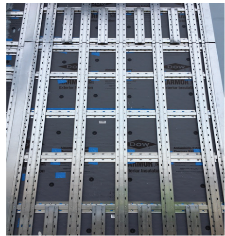
4. Vertical furring at 17-7/8" o.c. over horizontals. Additional vertical segments added to enable 9" o.c. Vertical Starter Track fastening. (Knight HCI™ System girts shown)
