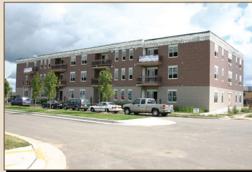
Apartments Front View During Construction
