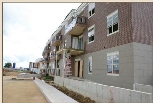
Apartments Under Construction
