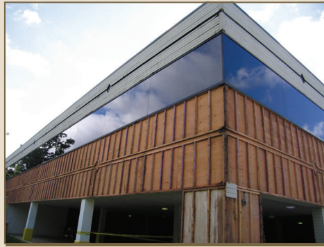
Tear off existing fiber board siding
