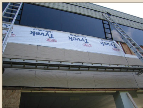
Installing Nichiha SandStone™ Panels
