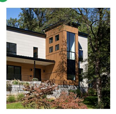
resist warping, rotting, pests, and fungi. Even in sub-zero temperatures, panels are highly resilient to cracking or buckling in freeze-thaw cycles. In either environment, cladding can tolerate winds up to 130 mph or higher and, in the event of a fire, will not combust, complying with even the industry's strictest safety codes.
